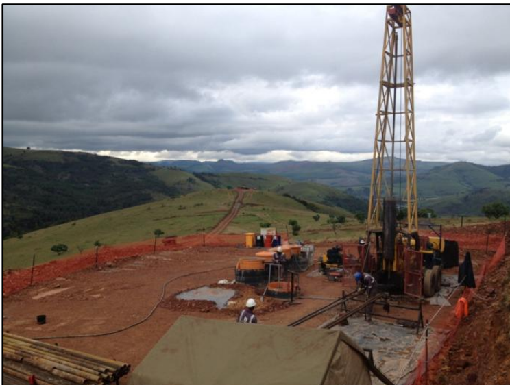
Drilling Borehole 14 showing the constructed road in the background
